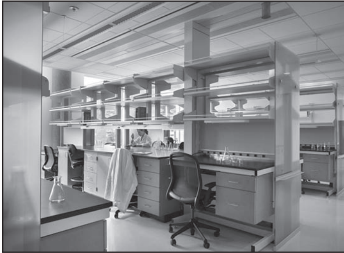
FIGURE 5: UW Medicine Phase 2 finished lab with chilled beam placement directly above the lab benches. (Photo courtesy of Ben Benschneider.)
